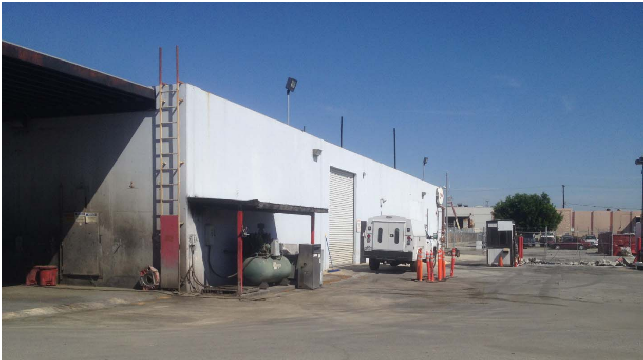
FIGURE 7. SOUTH SIDE OF BUILDING
