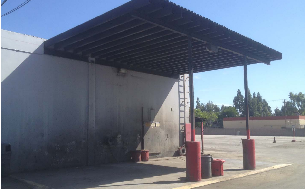
FIGURE 6. WASH BAY ON WEST SIDE OF BUILDING
